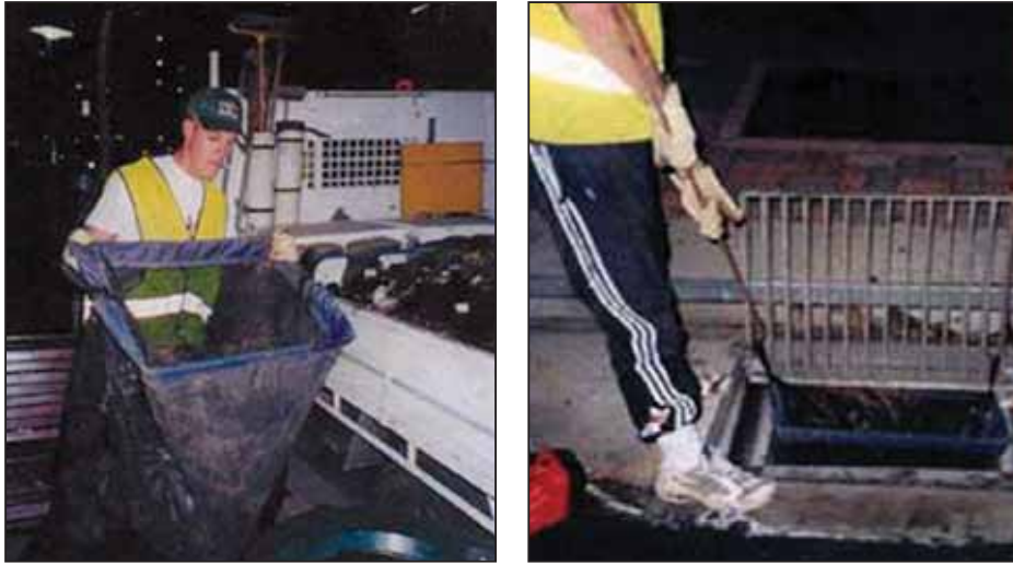
Plates 5.1 and 5.2 The Bag Liners Used in the 'Enviropod' Side Entry Pit Traps (photos courtesy of Ingal Environmental)
