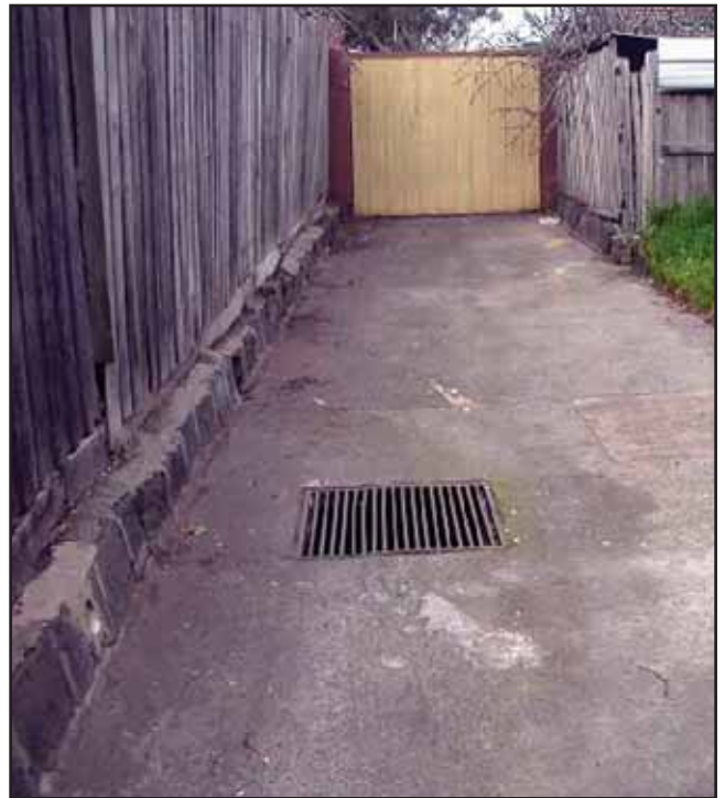
Plate 4.2 Cleaned Laneways Behind the Traders' Premises at Snell Grove (Observed During the Second Baseline Survey)
